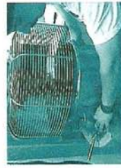
Machinery is guarded with a metal cage to protect the worker.
