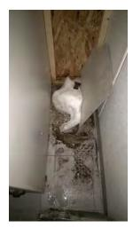
Snow in a transmitter building is a sad thing. Due to improper installation, the HVAC unit at the transmitter site serving Laramie and Cheyenne allowed snow to enter the building. This has caused significant outages during the end of May and beginning of June. WyomingPBS continues to replace damaged parts.
